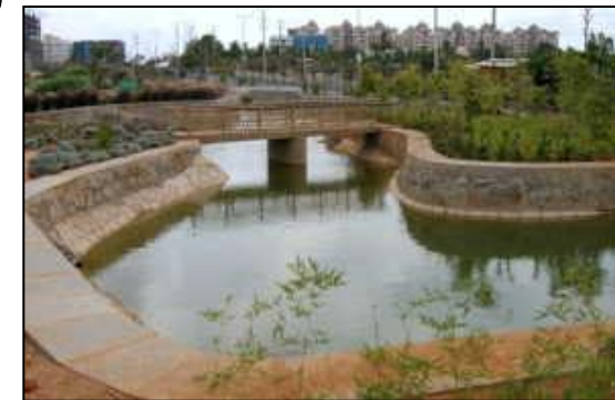
Rain water harvesting Pond
