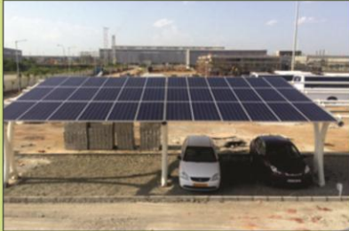
Danfoss Industries Pvt Ltd - Production Buildings Chennai - IGBC Platinum
