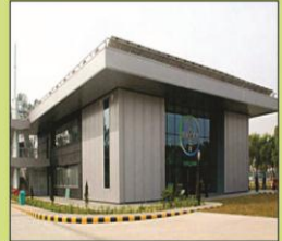
Eco Commercial Building, Noida - IGBC Platinum
