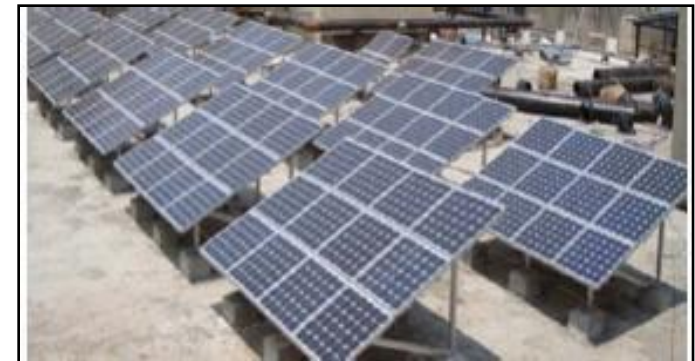
Installation of Solar PVs
